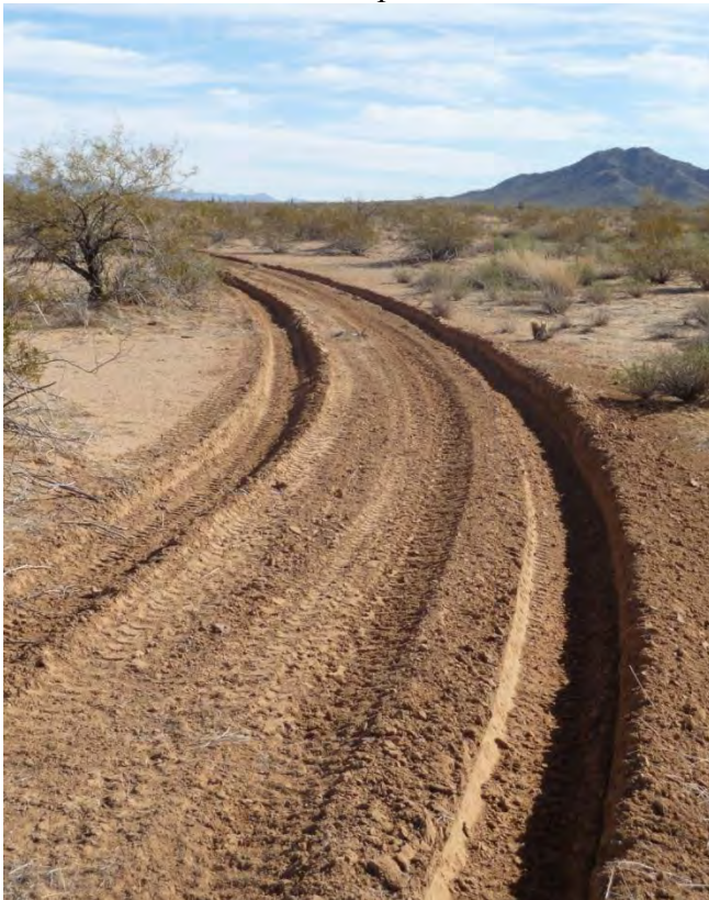
Class 3 - Soil berms built up around tire tracks. Disturbed soil and no vegetation between tracks
