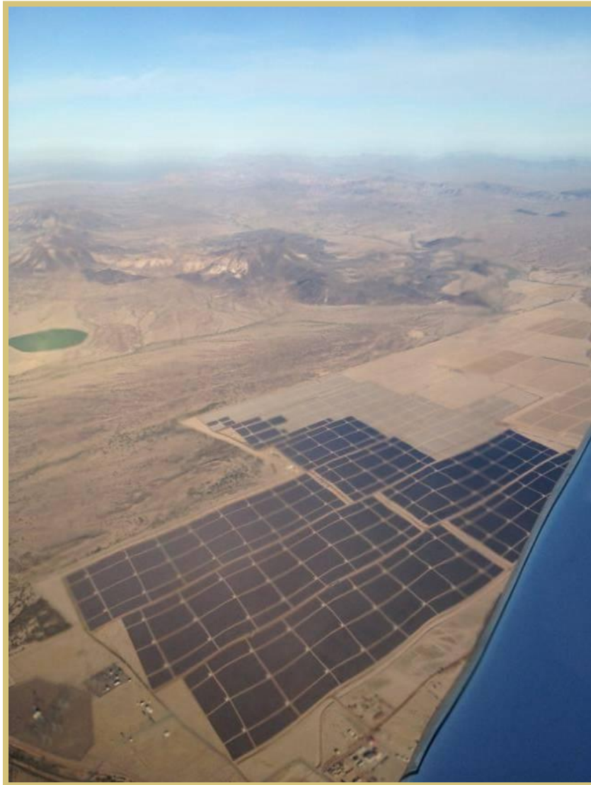
Figure 1: Photovoltaic solar site on private land adjacent to the proposed Agua Caliente SEZ. © Dave Richins
