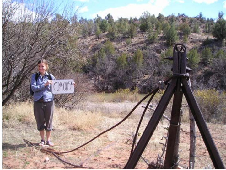
Photo CM-0054: Cable across river, leading to this short, steel tripod
