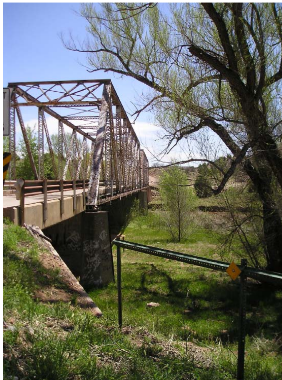
Photo CM_26a: Perkinsville Bridge crossing Verde River
