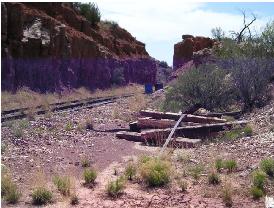
Photo CM_17a: Railroad ties near railroad grade, ~1 mile upstream of Perkinsville Bridge
