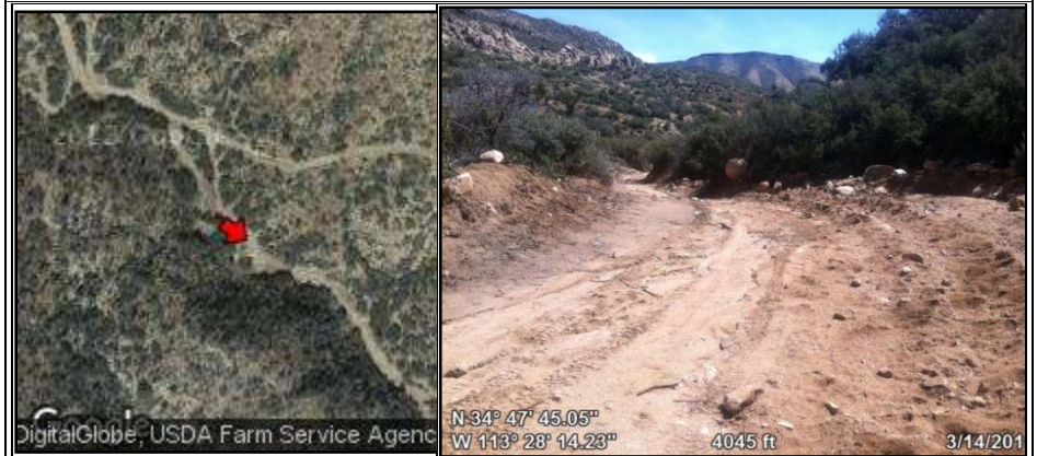
Photopoint 038. This cherrystem road has received very recent maintenance.
