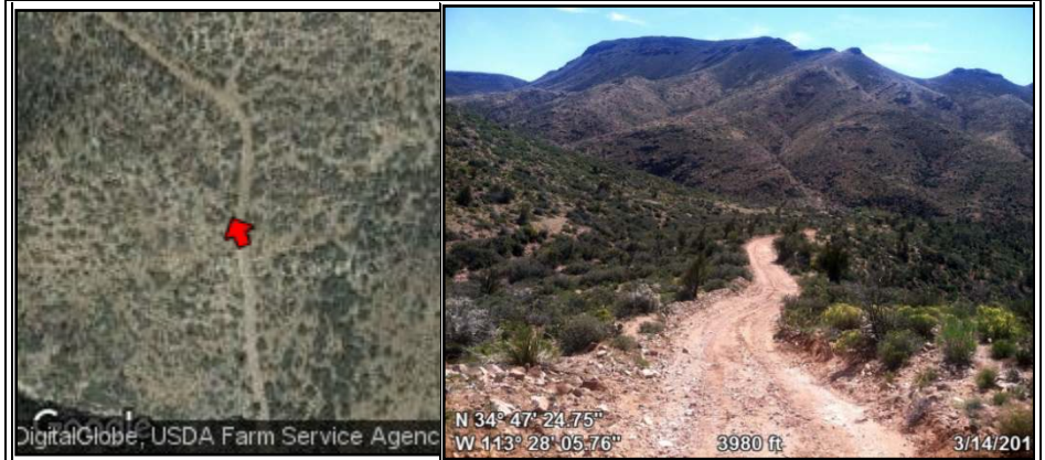
Photopoint 039. Roadside berms indicate recent maintenance.
