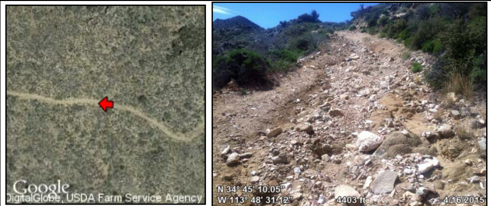
Photopoint 215. An extremely eroded hillside on BLM Route 7252 which leads to abandoned mine projects which are now revegetating.
