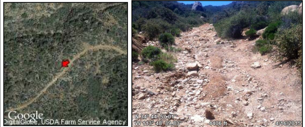
Photopoint 214. Erosion is evident along BLM Route 7334, but the route is excluded because it leads to private land and it is an impact to naturalness.
