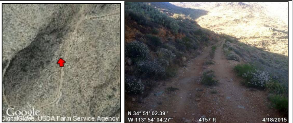
Photopoint 078. Vegetation in median indicates a lack of mechanical maintenance.
