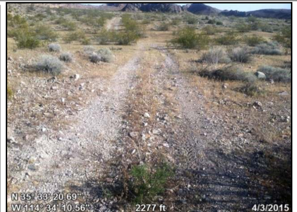
Photopoint 096. Perennial vegetation growing in median indicates a long-term lack of mechanical maintenance.
