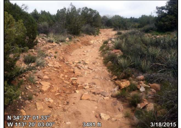
Photopoint 016. Evidence of erosion and a lack of maintenance on this section of BLM Route 7541.
