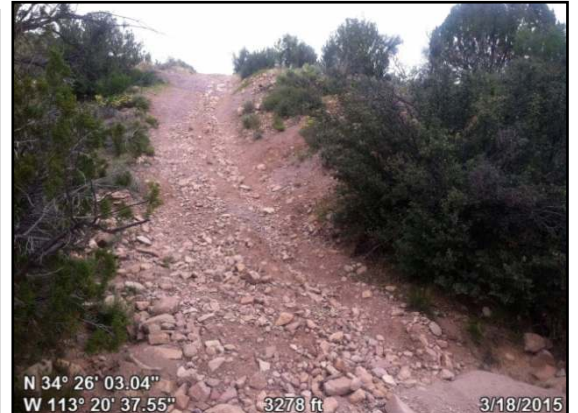
Photopoint 018. Much of the route is badly eroded, unsustainably steep, and only the width of an ATV. Where the route parallels washes it is significantly off-camber, indicating that it had never been mechanically constructed, or all evidence has naturalized due to having never been maintained.
