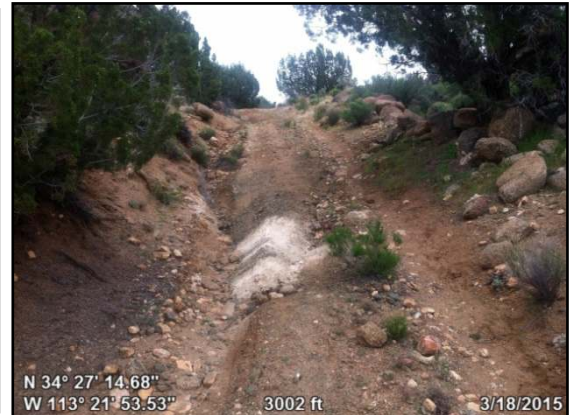
Photopoint 010. Erosion indicating a lack of maintenance on the way seen in Photopoints 8 & 9.
